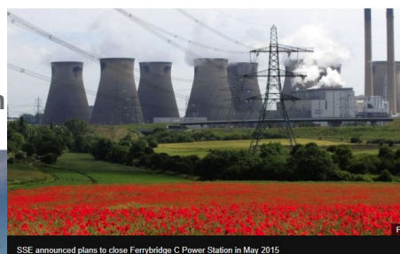
SSE announced plans to close Ferrybridge C Power Station in May 2015
