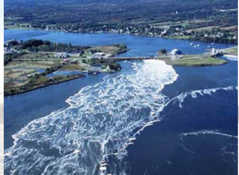
Annapolis Royal tidal barrage, Canada (20 MW)
